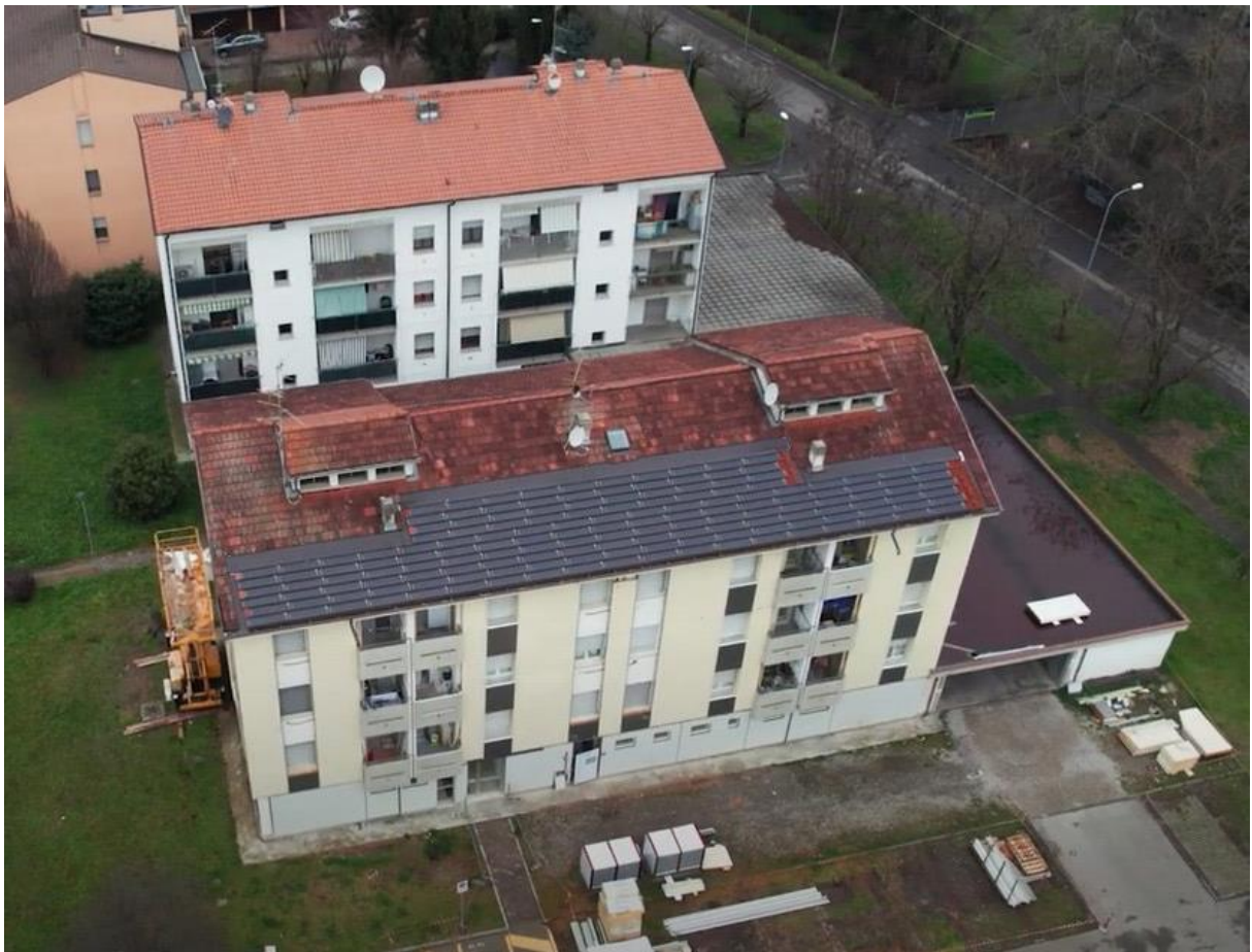
Installation of a 10 kW p SOTTILE system
